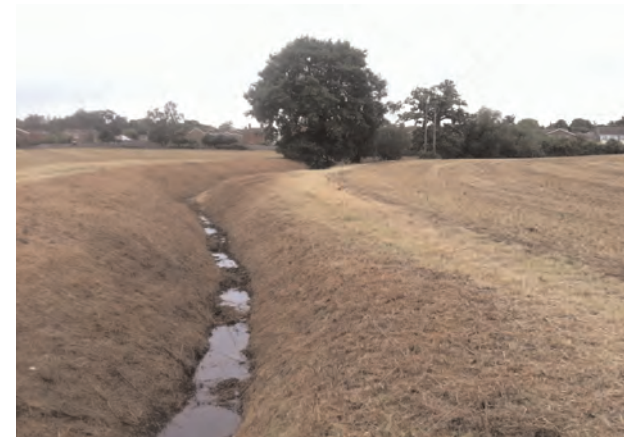
Figure 4.4 Drainage Ditch looking North
