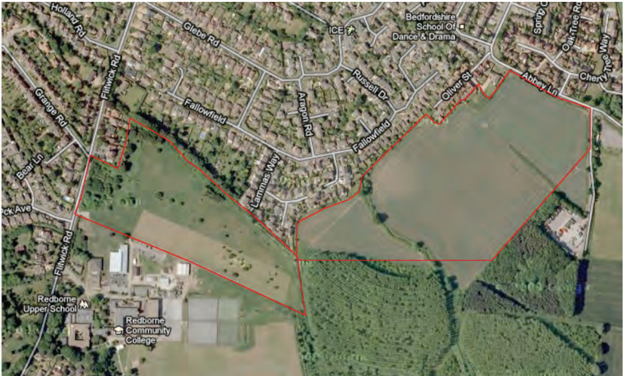
Figure 1.1 Warren Farm Amphill: Aerial Photograph showing site allocation and boundary
